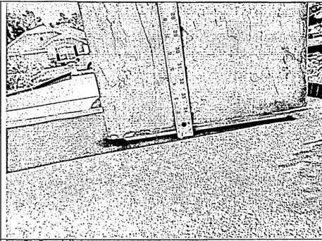
23. Issue: A weeping accessory must be present at any horizontal and vertical intersection to allow moisture to exit.
