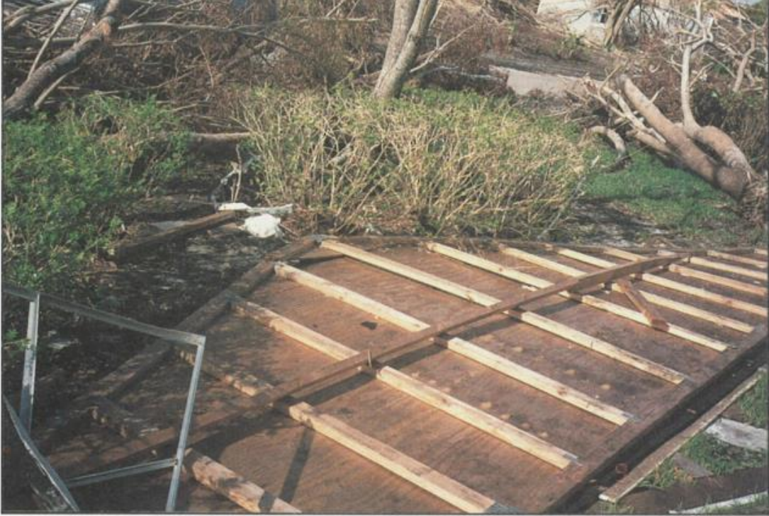
FIGURE 6. Entire wood gable separation. Bracing connection, if completed, may have prevented this from occurring.
