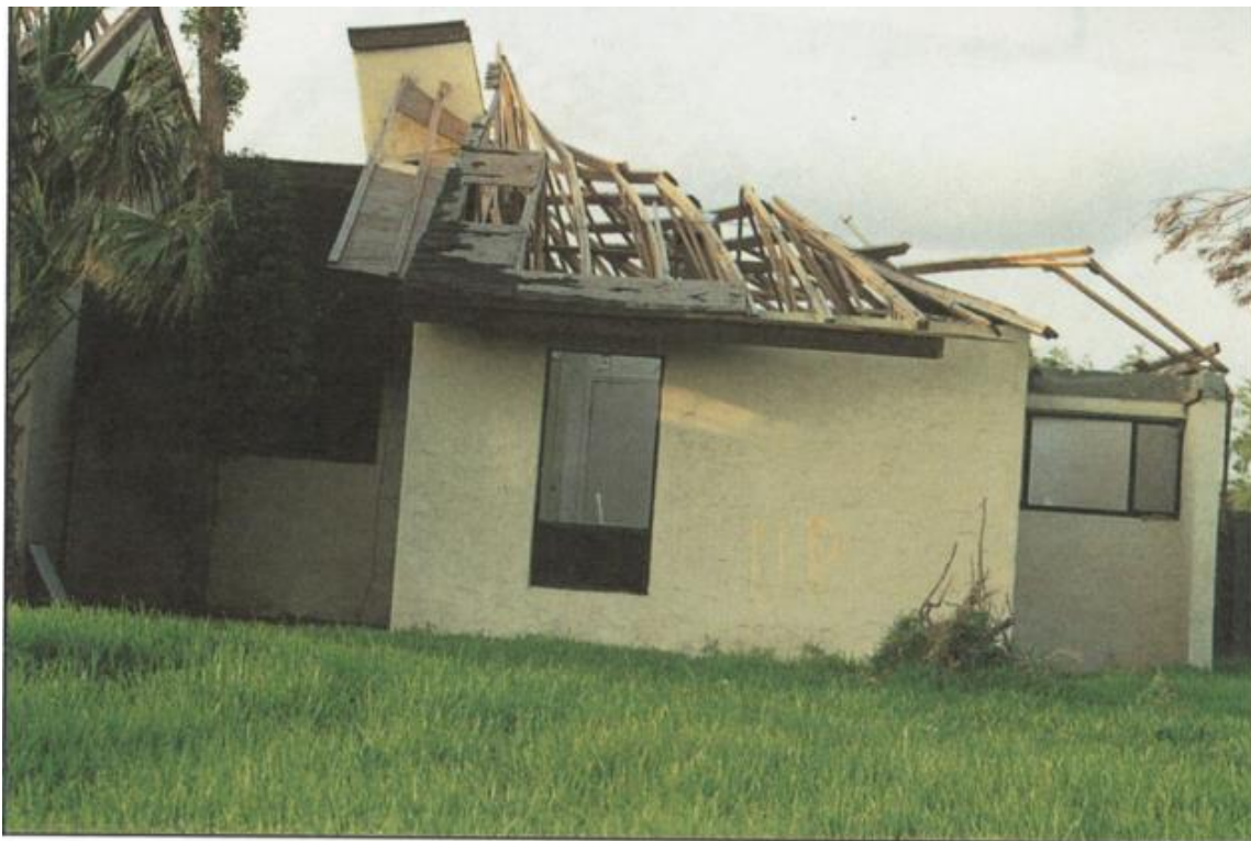
FIGURE 14. Roof structure failure due to inadequate bracing.
