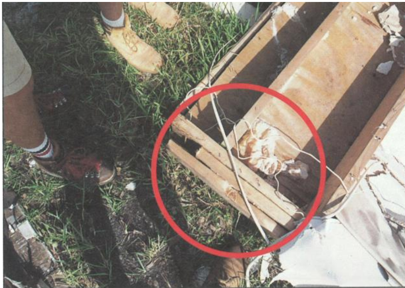
FIGURE 10. Top plate splice not able to transfer horizontal loads.
