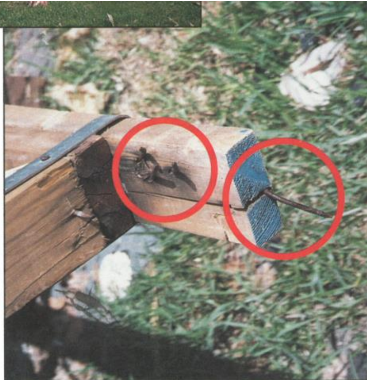
FIGURE 5. End of exterior non-loadbearing wall top plate. Transfer of forces on entire wall depended on a limited number of nails.
