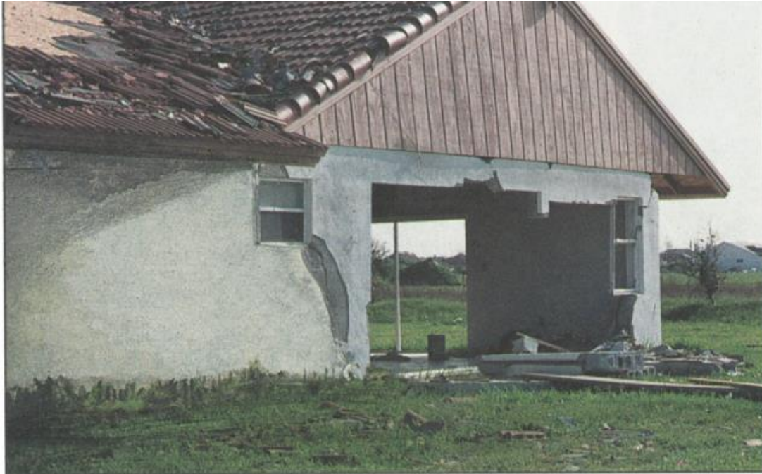
FIGURE 15. Masonry construction building. Wall separated from building envelope due to inadequate vertical wall reinforcing in connection to horizontal tie-beam.
