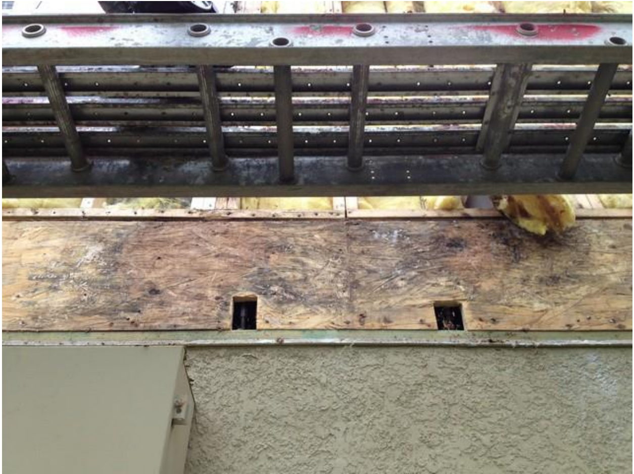
Stucco and wood removed from the exterior of this KB Home due to water intrusion damage.
