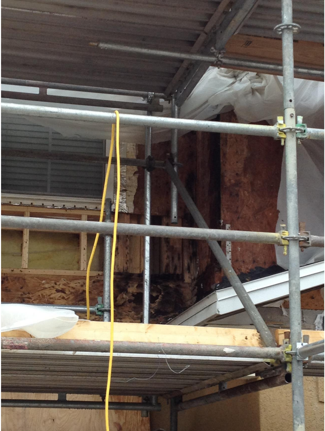
Once stucco was removed, rotted wood was revealed on this KB Homes exterior.
