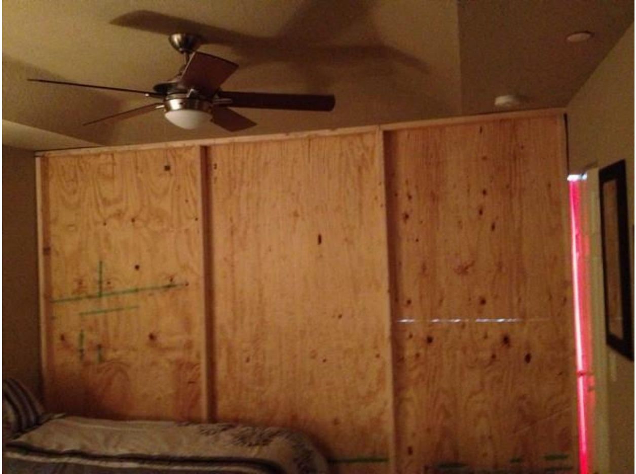
This is the wall barrier that is set up inside KB Homes Willowbrook homes to separate homeowners from the massive amount of construction work needed to totally reconstruct their balconies and alleviate water intrusion issues.
