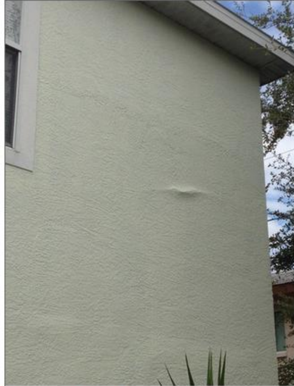
Signs of water intrusion on exterior of KB Home Image 6 of 20 < Prev Next >
