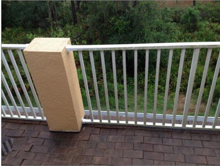
Can you see the guiderail bowing in? This KB Home exterior balcony is failing Image 17 of 20 < Prev Next >
