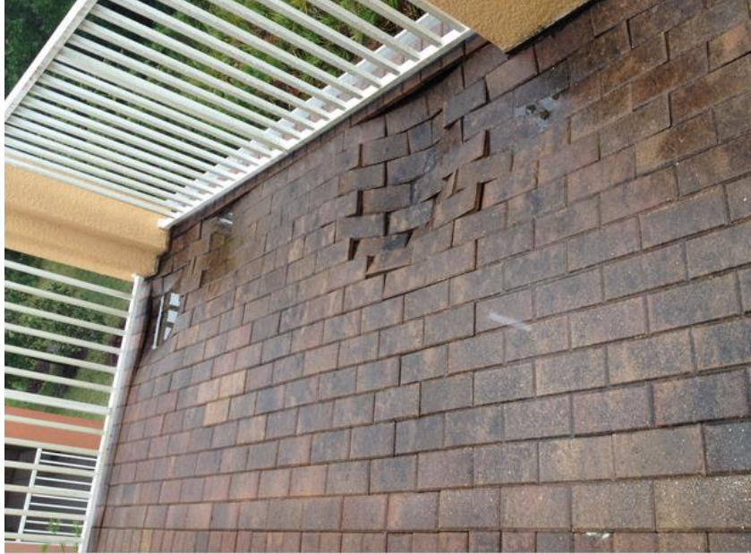
During a rain, you can see the water pooled up in this KB Homes balcony that has failed. Homeowner hasn't stepped foot on this balcony in over 16 months.
