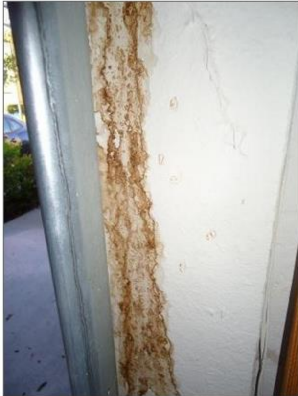
KB Homes water intrusion, mildew and mold in garage from water intrusion on front of building. Image 17 of 20 < Prev Next >
