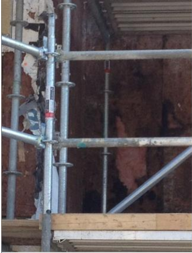
More stucco and rotted wood removed from KB Homes Willowbrook townhomes, getting to the source of water intrusion
