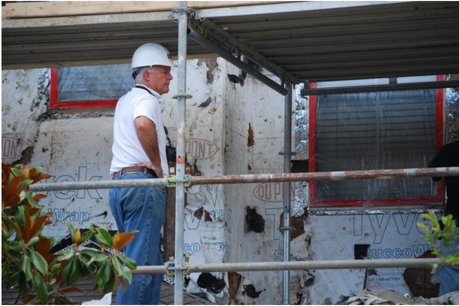
More stucco and rotted wood removed from KB Homes Willowbrook townhomes, getting to the source of water intrusion
